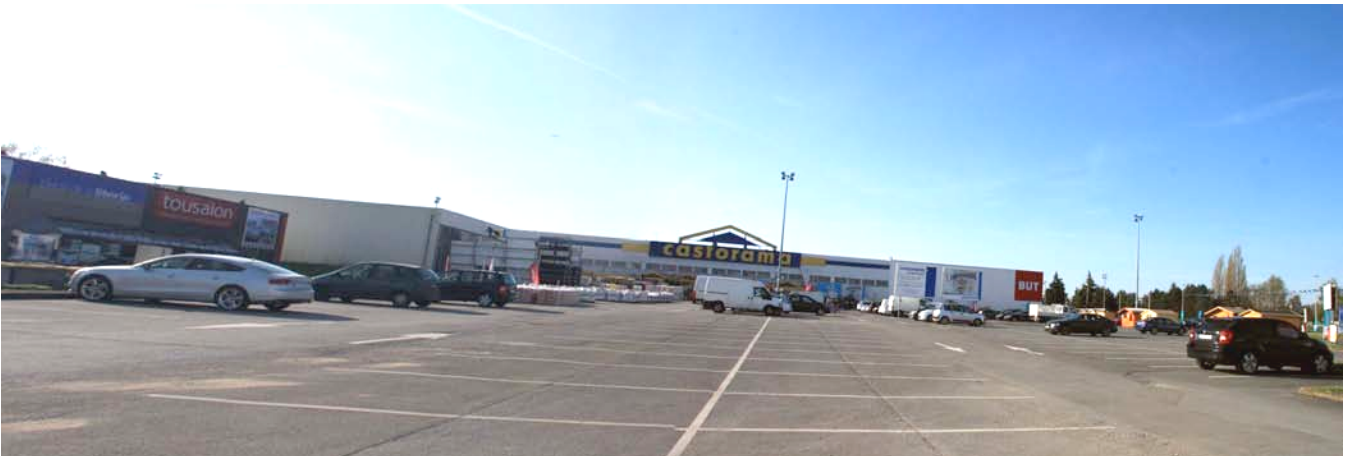
4 – Vue parking nord
